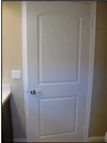
Interior Wood Door
